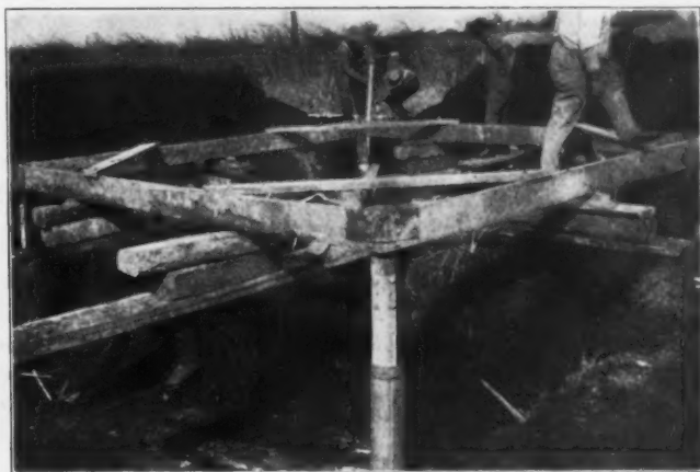
FIG. 23—EXCAVATION FOR FLOATERS, CICERO SWAMP
